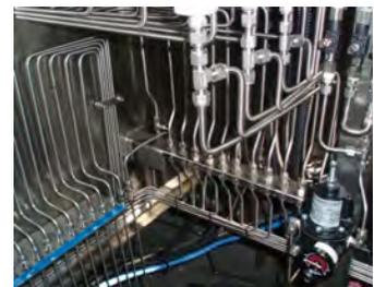
above-listed products packaged in a stainless steel control panel built at Altronic Controls. The installation presented Chevron with a turn-key controls retrofit and mechanical overhaul. Quimex S.A. specified the mechanical scope and controls upgrade scope in its entirety and provided the control panels and complete set of end devices, installation materials, installation tooling, and all mechanical overhaul parts required for the project.
