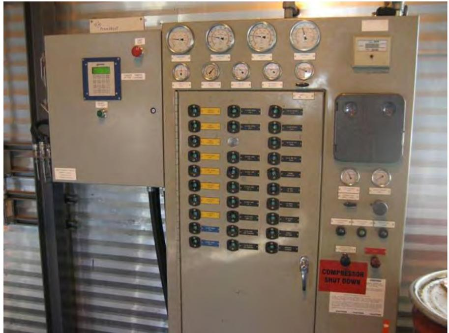
*Existing pneumatic control panel with compact DE-3000 panel mounted on left side.*
