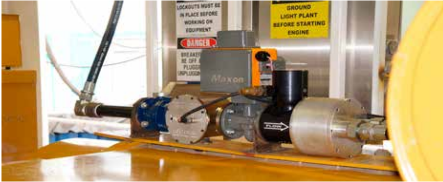
Typical Flanged Gas Train Assembly
