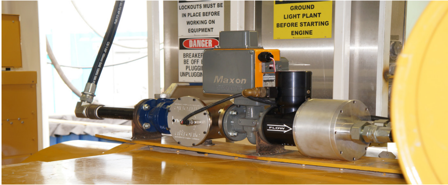
Typical Flanged Gas Train Assembly
